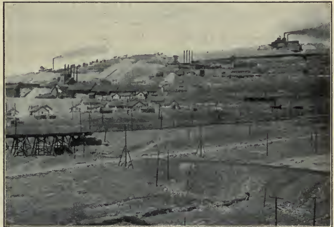
FIG. 290.—A view in the mining district of Victor, Colorado. There are mines beneath these buildings, and the waste rock removed from the tunnels forms huge banks near them.
